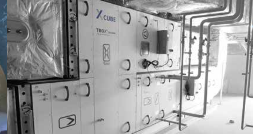
21 X-CUBE air handling units provide the museum with 130,000 m³ of conditioned air per hour. (Picture: TROX)
